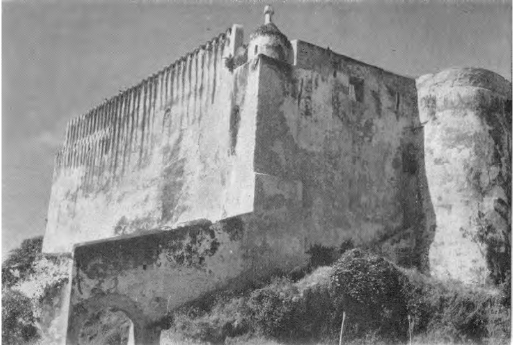
Portuguese workmen started raising the high walls of coral rock almost a century after Vasco da Gama had dropped anchor of Mombasa on his way to India.
